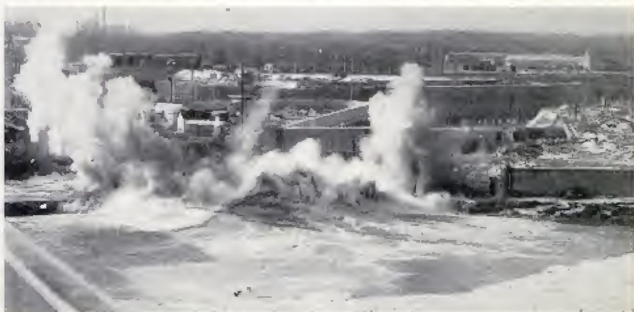
Huge wave was created by blast, but air curtain absorbed shock waves. Only a tremor was felt at powerhouse. Below, rock barrier was completely shattered by massive charge of explosives. Cost of project was $2000
